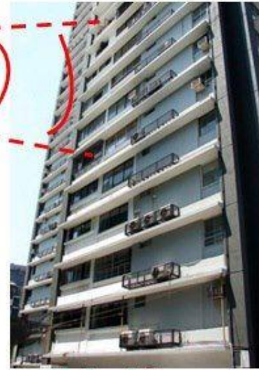
Usha Kiran Building
